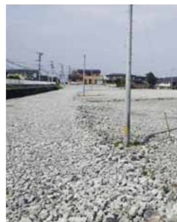
Road using PAMCO Crushed Stone roadbed material
