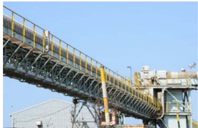
Raw material conveyor: Raw material conveyor is total around 2.4km length.
